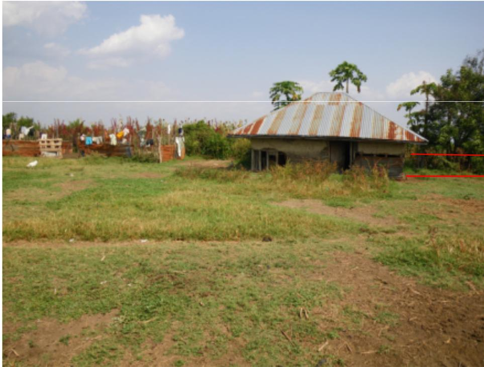
The wall of house was soaked by flooded water and collapsed. Depth of flood water was estimated as 80 cm by flood mark.
